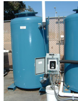
Model 112 at Gas Station Monitoring Carbon Bed Outlet
